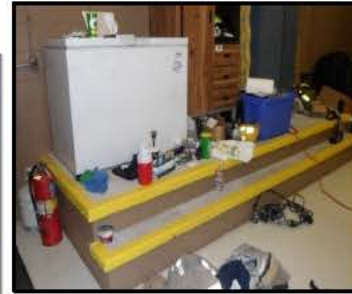
Example of Raising Utilities above Design Flood
